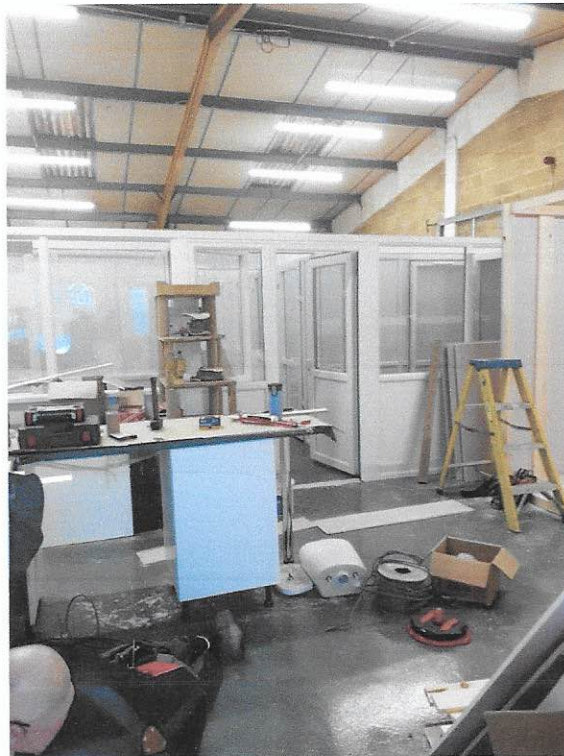
Work in progress at the Apsley Cattery
